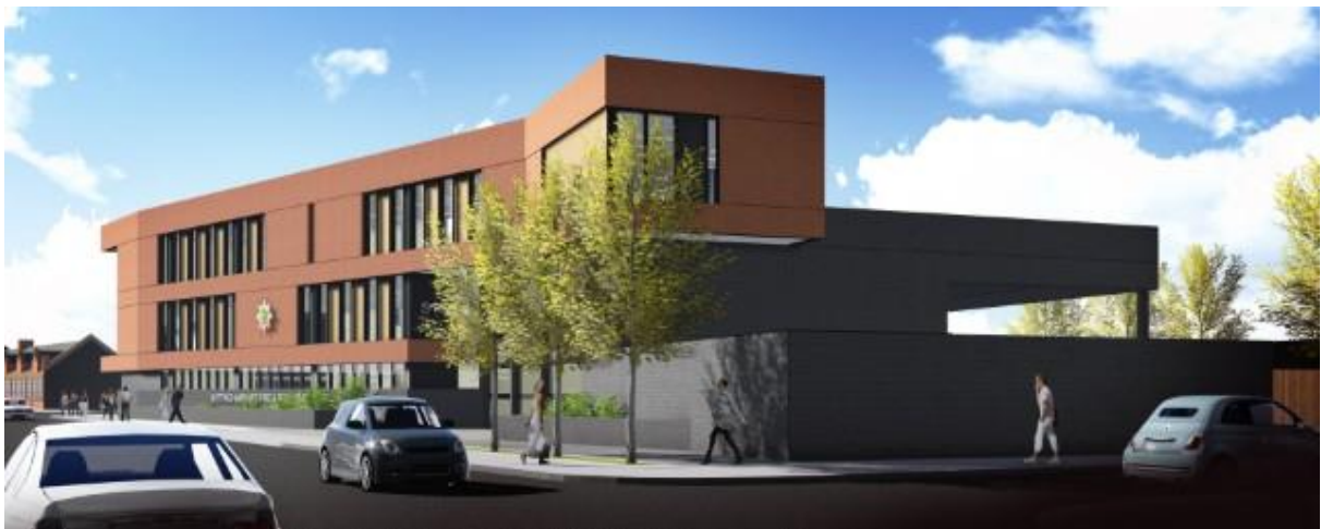
View down London Road towards Trent Bridge
